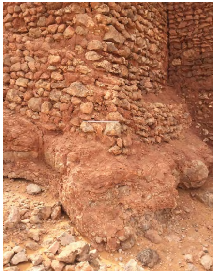
Fig. 6- Semjane, construction detail of corner tower with the Hamada rock (Illili Mahrouf, 2015).
