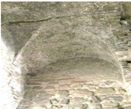
Fig. 12- Cross-vault above the gateway entry (Abdessemed-Foufa, 2016).
