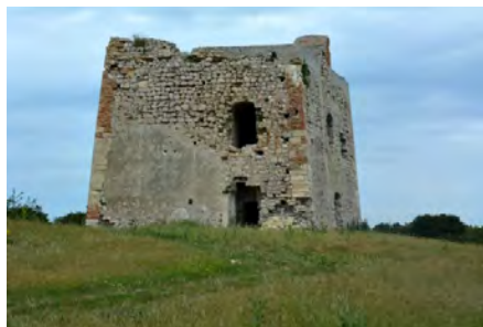
Fig. 2- The tower from the lake side.
