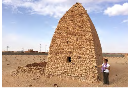
Fig.5- Unlimed stone mausoleum and the cemetery of Sidi El Hadj Lahcen in Guentour (Illili Mahrouf, 2015).
