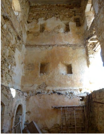
Fig. 9- Tower-house in Giannoudion, interior east elevation (section AA' in Fig. 8) (Emma Maglio, 2014).
