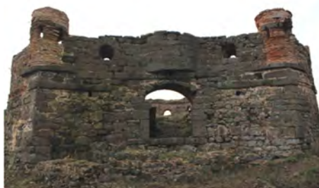
Fig. 3- North façade of the late 18 th century Garipçe Tower.
