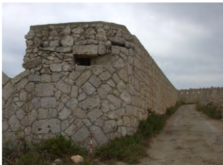
Fig. 10- PD2: all perimeter defences have at least one MG opening and one observation opening.
