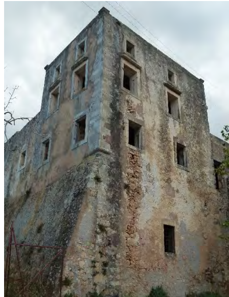
Fig.3- Tower-house in Mikro Metochi (Emma Maglio, 2014).
