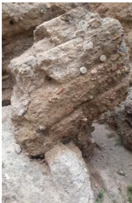
Fig. 6- Reinforced earthen walls with logs of tuya (Abdessemed-Foufa, 2016).
