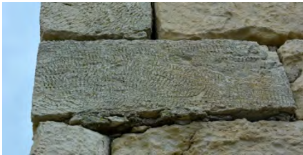
Fig. 8- Toothed chisel traces on stone blocks.
