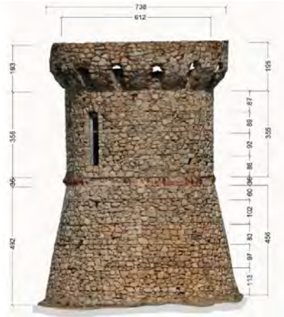
Fig. 10- Tower of the Isolella, survey of the mass volume with the photogrammetry program Autodesk 123D Catch (Casu, Pisu, 2013).
