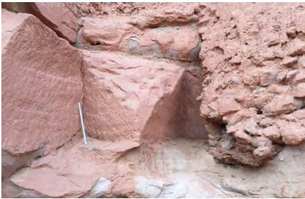
Fig.11- Aghem Taouersit. Tooling traces at foot perimeter wall (Illili Mahrou, 2015).
