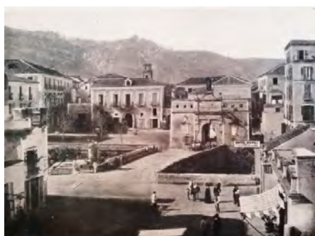
Fig. 6- De Luca, The castle square , 1860 ca. The image shows the square after the demolition of the castle (Filangieri, 1929).
