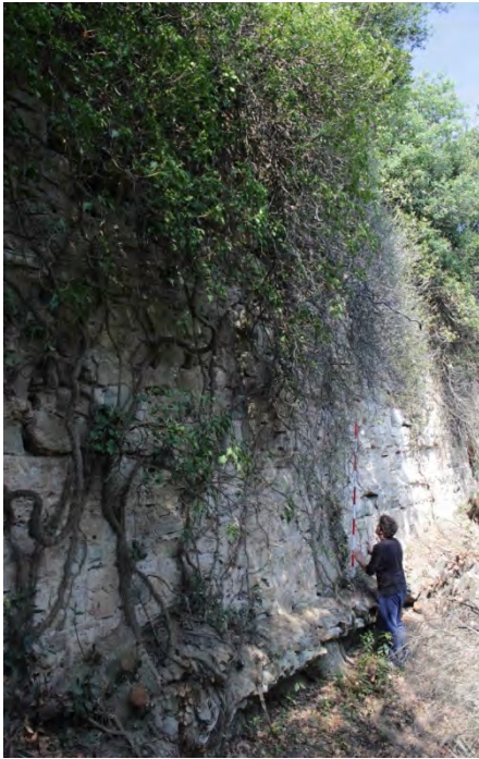
Fig. 9- South walls of the Upper Rumeli Kavak fortress.
