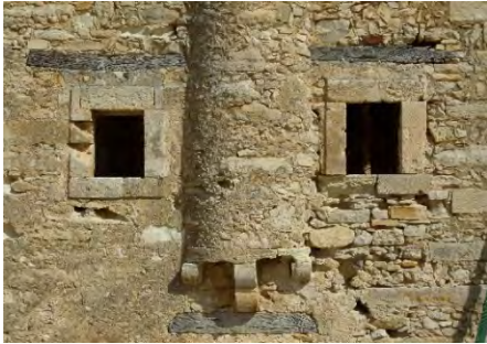
Fig. 7- Tower-house in Giannoudion, west elevation, detail (Emma Maglio, 2014).
